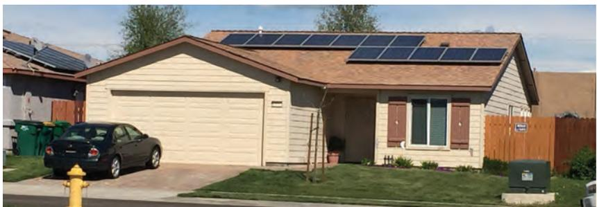
GTI began efforts on a California Energy Commission project to demonstrate the potential of ZNE homes that generate as much energy as they consume. GTI is developing and testing advanced energy efficiency packages using low-cost construction methods, high-performance housing techniques, and solar PV in two identical homes: one all-electric and one mixed fuel. The project is being conducted with Habitat for Humanity in a new affordable housing community in Stockton, California.
