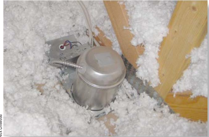
**Fig. 2.9 Modern air-tight, IC-rated can light**
