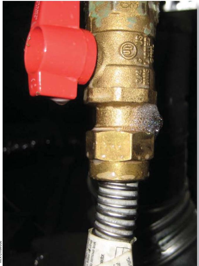
Fig. 5.14 Detergent solution - Visual gas leak detection
