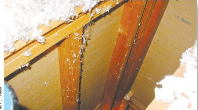
Fig. 9.4a Open soffit, above bathroom closets
