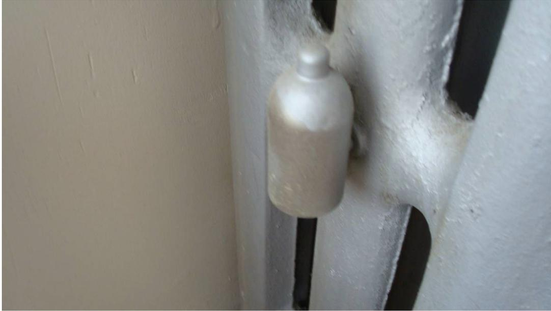
**Figure 7. Painting over radiator vents is a common oversight that can have a serious effect on the heating in an apartment. Blocked radiator vents must be replaced.**
