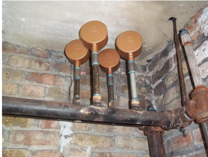
**Figure 5. Main line air vents installed on a steam line.**
