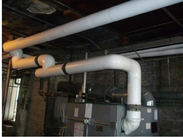
**Figure 8. Insulated heating pipes**
