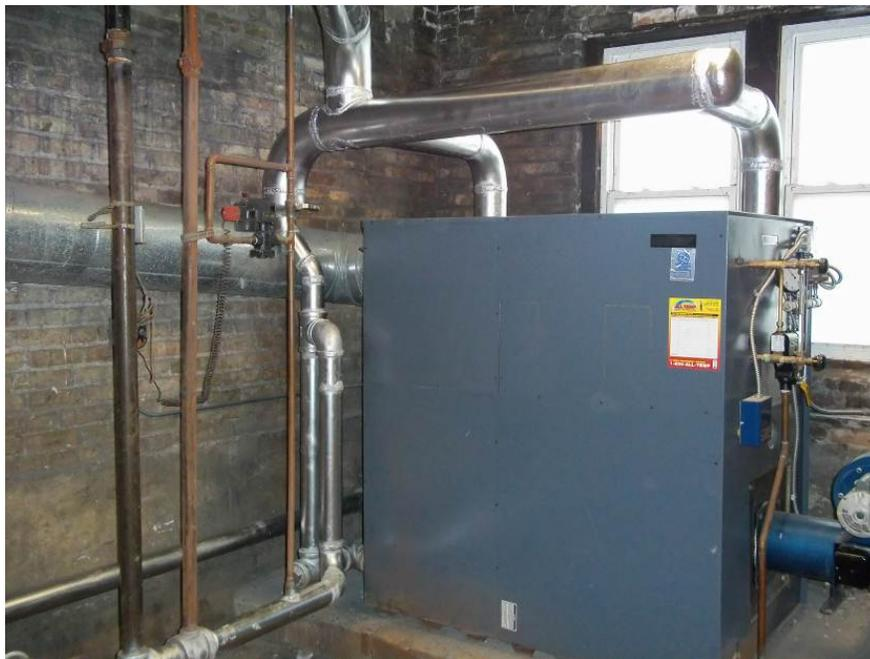
**Figure 2. A cast-iron sectional steam boiler in good working condition in a building that could benefit from balancing**
