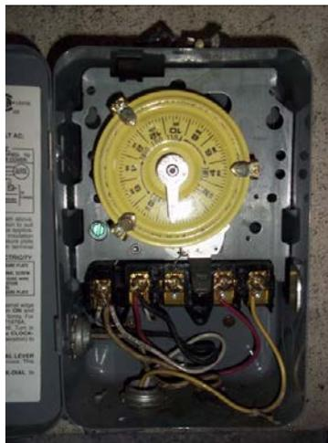
**Figure 9. Time clock control for a steam boiler**
