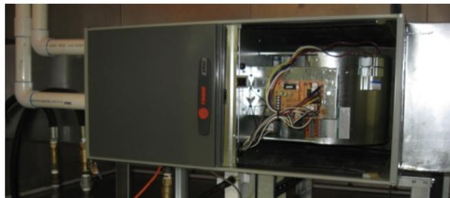
**Figure 9. Attic installations are typically horizontal left or right**
