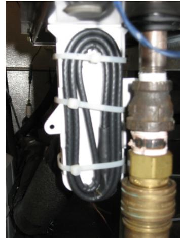
**Figure 5. Heat tape on a condensate trap**
