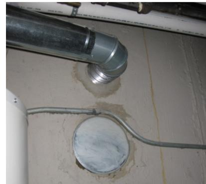
**Figure 13. Seal unused vent openings**
