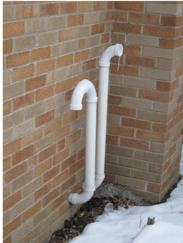
**Figure 12. Vent termination above the snow line**
