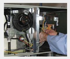
Adjust the airflow for the location by selecting a fan speed that produces an air temperature within the rise range specified by the manufacturer.
