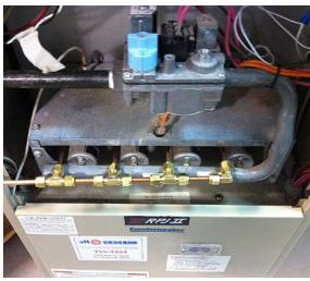
Laboratory testing requires the use of a tracer gas for atmospheric furnaces.
