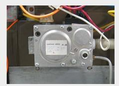
Tune the gas valve to set the firing rate at installation.
