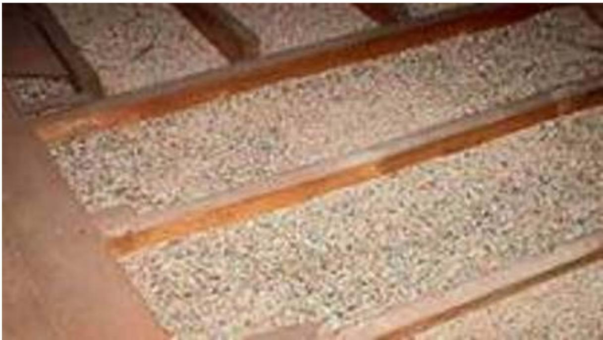
**Figure 2. Vermiculite insulation between joists**
