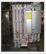
The tankless water heater delivers DHW and hot water to a fan coil (hydronic furnace) for space heating.
