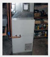
With minor duct transitions, the hydronic furnace was a simple replacement for the existing furnace.
